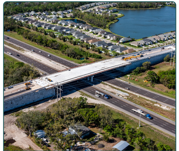
Southwest-facing view of construction of the bridge over I-75
