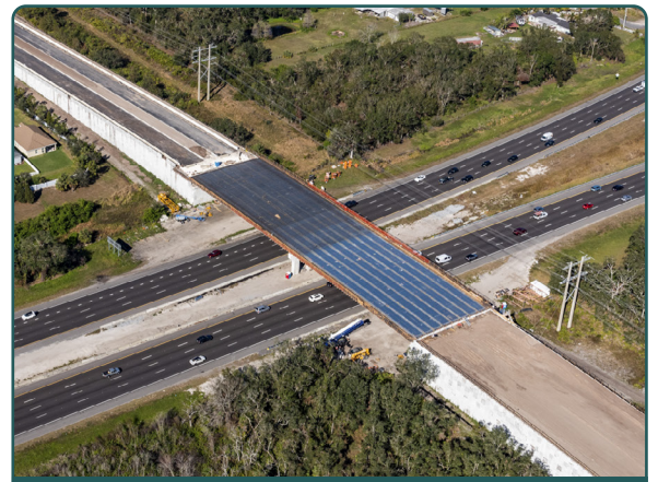
Northwest-facing view of bridge construction over I-75
