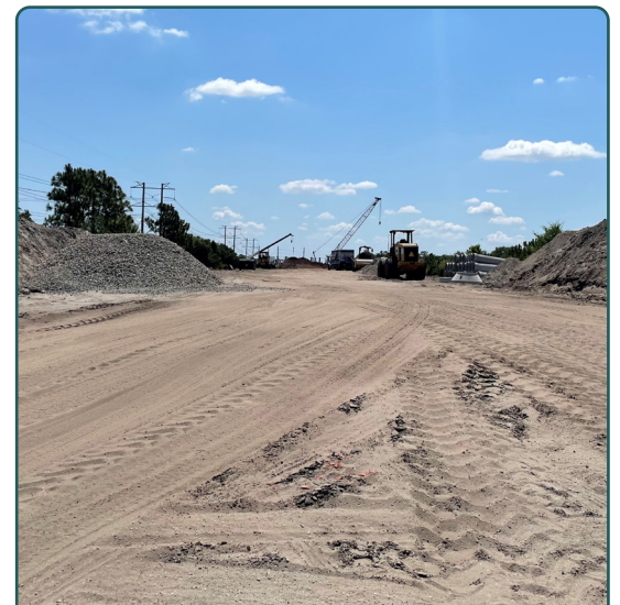
Eastern view of construction from west of I-75
