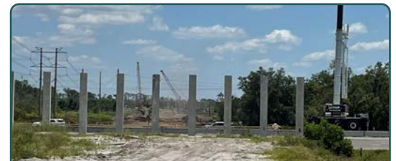
Eastbound view from future western bridge approach over I-75
