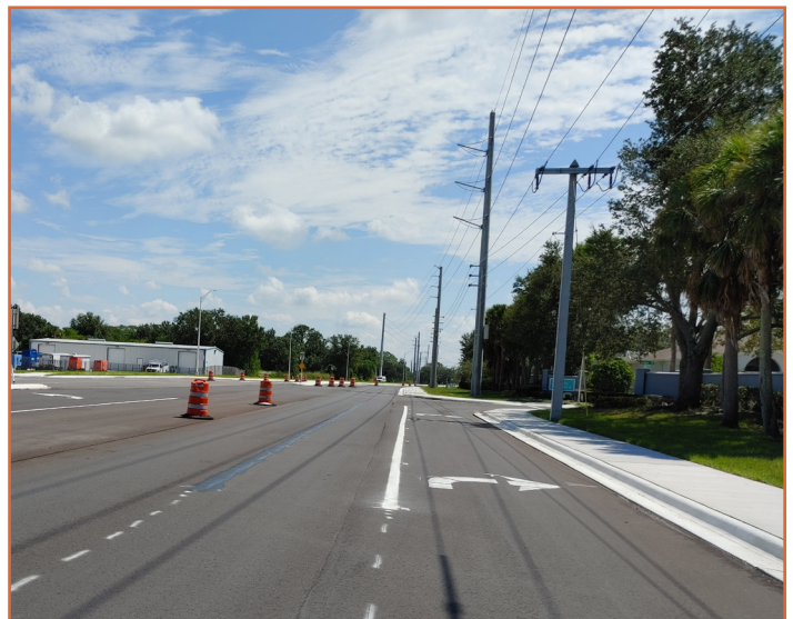
Temporary pavement markings in place in preparation for permanent markings
